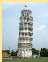
Leaning tower of Pisa
